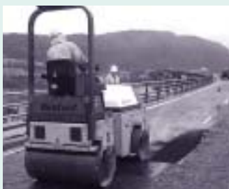
A90 Friarton Bridge surface patching
