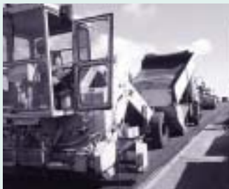
A90 Longhaven surface dressing
