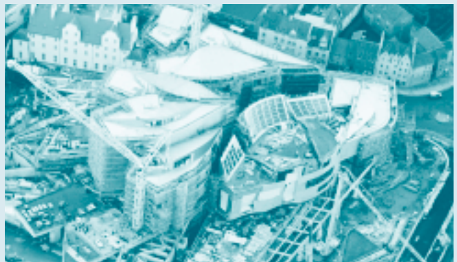
Main building complex (looking from south)
