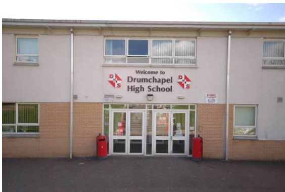
Low-key entrance only signified by signage
