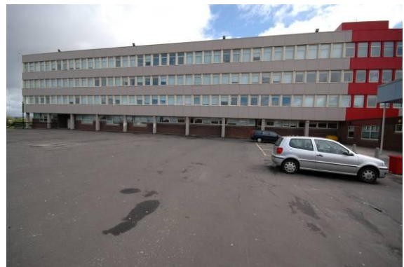
Extensive tarmac foreground to school entrance
