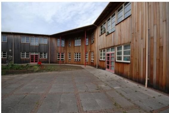
Cedar cladding to a school extension
