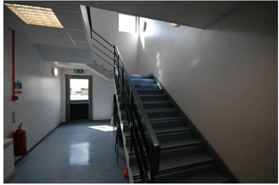
Restricted headroom – less than 2 metres
